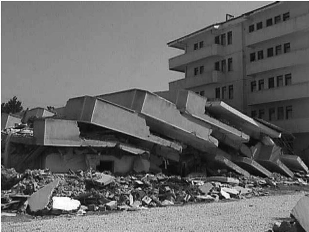
The photo, taken following the 1999 Izmit earthquake in Turkey, suggests that steel reinforcement in concrete columns and at junctions with floorslabs offered inadequate resistance to earthquake motion and to the load upon them. The collapsed floors remained largely intact. (Mehmet Celebi)
